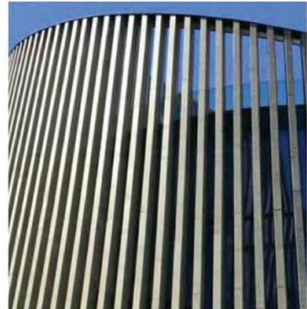
FIX VERTICAL TIMBER BATTEN
